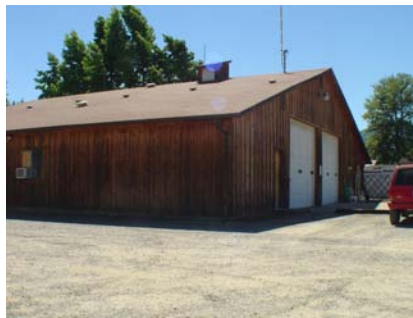
NE General Site Also shows garage doors are on both sides indicating that there is no torsion problem.
