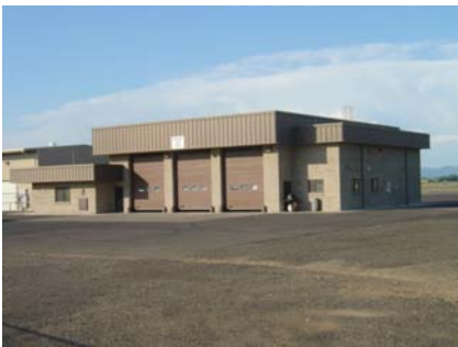
SW Elevation View also shows vertical irregularity, reentrant corner, and out of plane lateral system.
