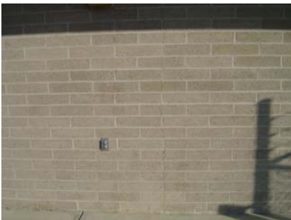
N Poor Condition There is a crack going from the bottom to the top cutting through the masonry.
