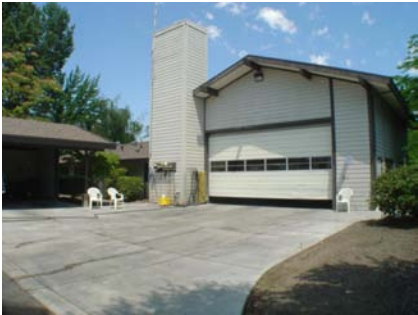
SE Elevation View Vertical irregularity due to the hose tower.
