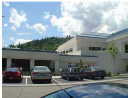
N Vertical Irregularity Primary Vertical Irregularity due to new building.
