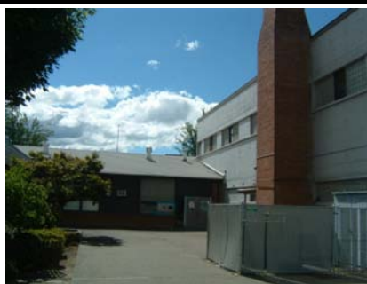
S Vertical Irregularity Primary also shows reentrant corner
