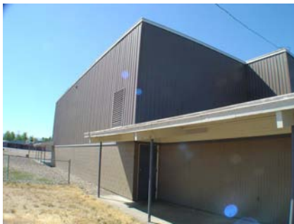
N Vertical Irregularity Primary also shows two lateral systems.
