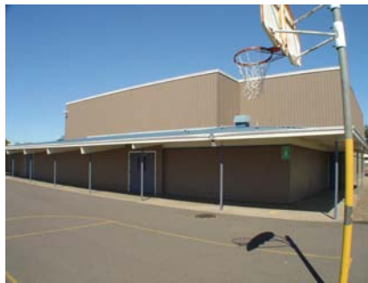
NE Vertical Irregularity Primary also shows out of plan irregularity.
