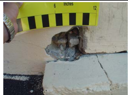
N Poor Condition There are some chunks of the building missing like this one.
