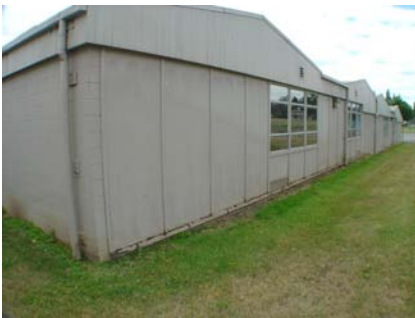
NE Elevation View shows a RM wall on the left and a W2 wall on the right.
