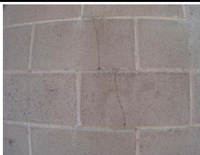
S Poor Condition There are cracks all over.
