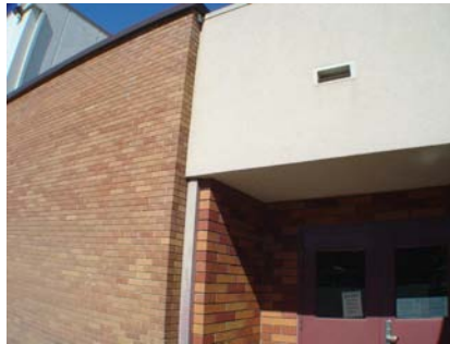
W Plan Irregularity Secondary Joint to newer building
