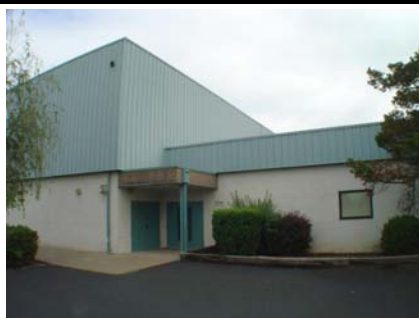
SE Vertical Irregularity Primary also shows reentrant corner.
