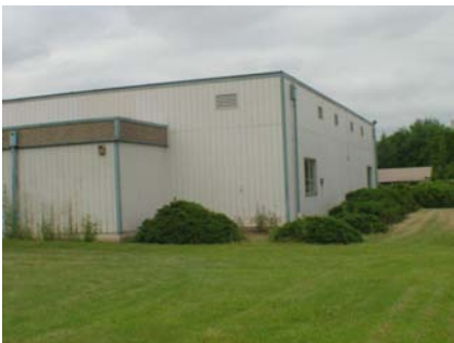
NE Elevation View also shows reentrant corner and elevation step.
