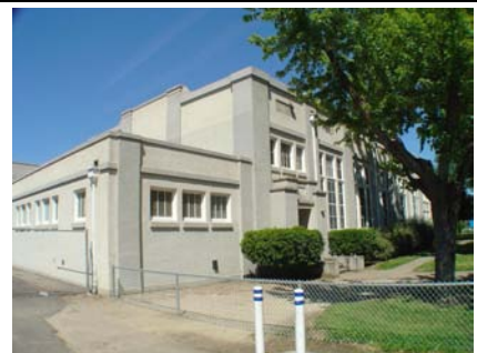
SW Vertical Irregularity Primary
