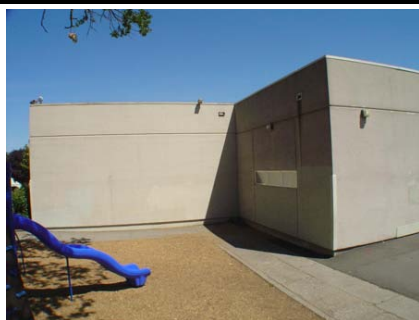
NW Plan Irregularity Primary
