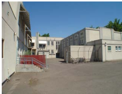
W Plan Irregularity Primary and plan irregularity: reentrant corner due to adjacent building.
