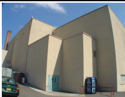
NW Elevation View elevation step and reentrant corner.
