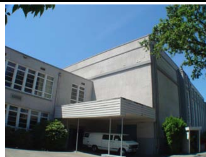
NE Vertical Irregularity Secondary Also plan irreg.
