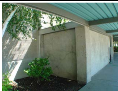
S Plan Irregularity Primary reentrant corner
