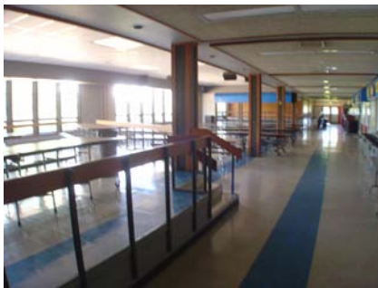
W Vertical Irregularity Primary Very large opening inside.
