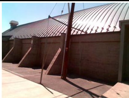
NE Elevation View
