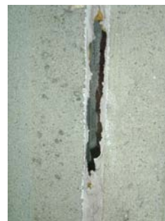
NW Primary Structural Type The masonry can be seen through this hole.
