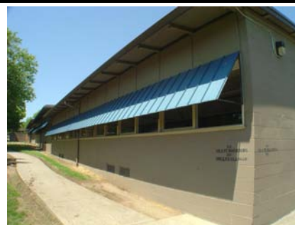
SW General Site
