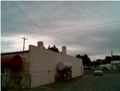
S Falling Hazard
