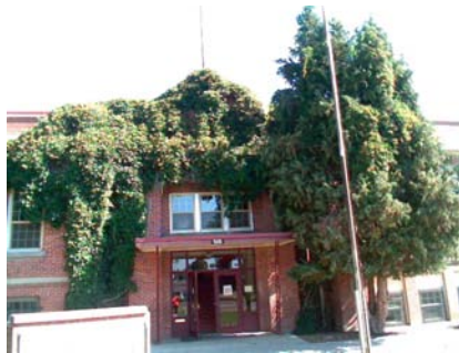
S Falling Hazard
