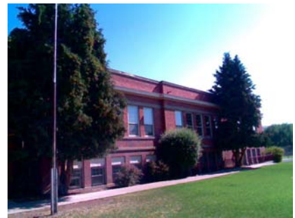
S Falling Hazard
