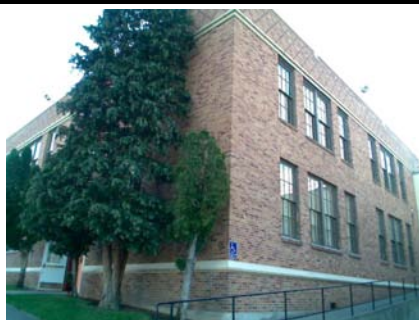
SW Elevation View
