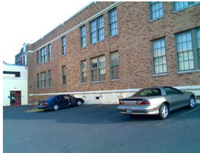
N Other seam showing addition
