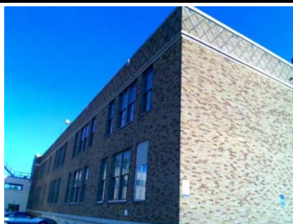
NW Seismic Upgrade
