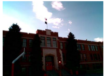
E Falling Hazard
