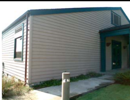
NW Primary Structural Type W2
