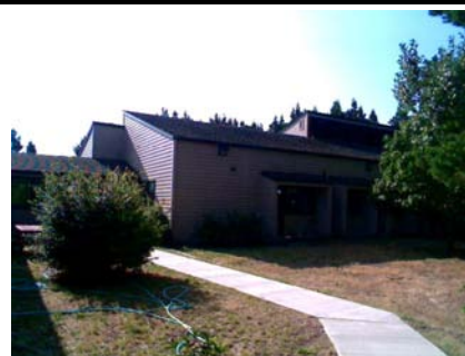
NW Plan Irregularity Primary Reentrant Corner and vertical irregularity.
