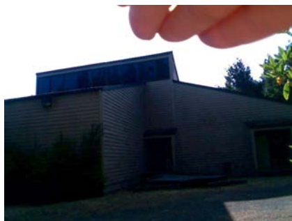
W Plan Irregularity Primary Reentrant corner and a vertical irregularity.
