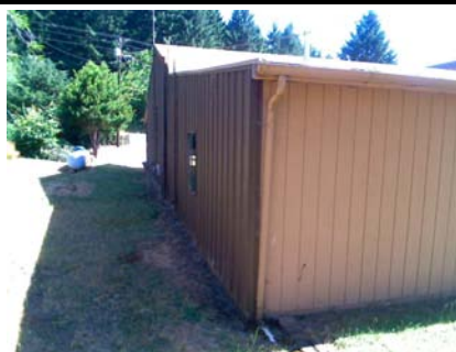
NE Primary Structural Type the east side of this building is sheathed with metal all other sides are wood.
