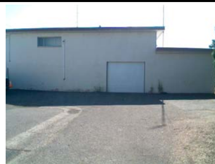
W Plan Irregularity Secondary shows an almost solid wall opposite the front wall which has large openings. Indicating possible torsion problems.
