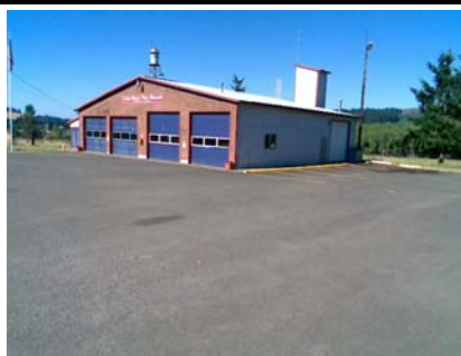
NE Plan Irregularity Secondary Large opening in the front of the building indicates possible torsion problem
