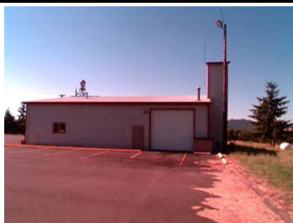
N Vertical Irregularity Primary Irregularity is due to hose tower
