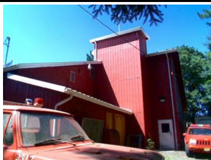
E Vertical Irregularity Primary also shows plan irregularity
