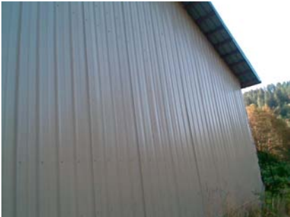
W Primary Structural Type back wall is solid - plan irregularity torsion.
