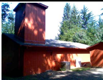
E Plan Irregularity Primary Back wall is solid indicating a potential torsion problem.
