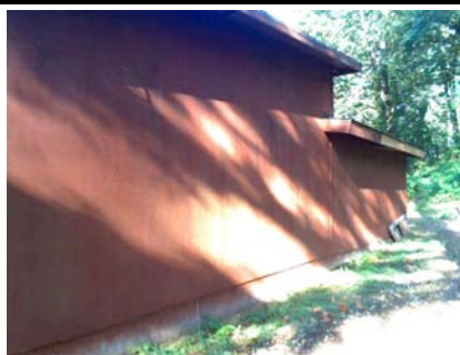
N Vertical Irregularity Primary Also shows the back wall of the building is solid indicating a potential torsion problem.
