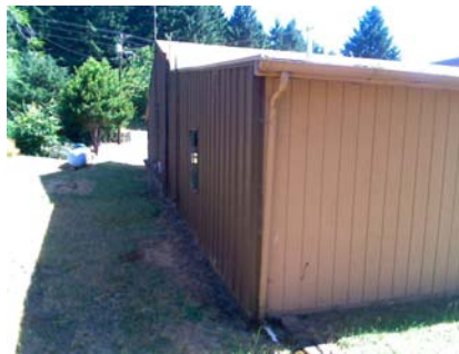
NE Primary Structural Type The east wall of fir76 is sheathed with metal sheathing (S3).
