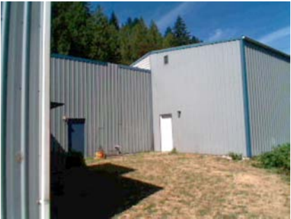
SW Plan Irregularity Primary also show elevation step.
