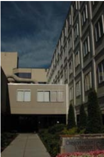
SE Vertical Irregularity Primary
