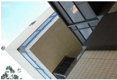
W Vertical Irregularity Primary cantilever portions
