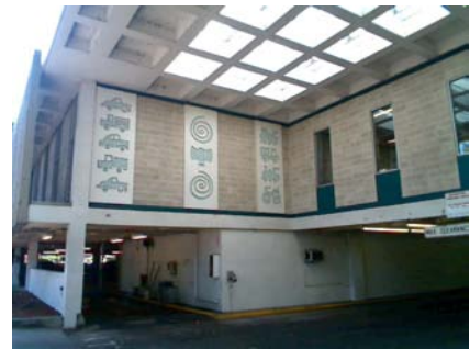
NE Primary Structural Type Tertiary structural type, also shows plan irregularity and short columns.
