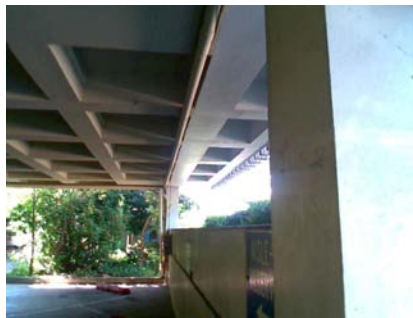
E Vertical Irregularity Secondary short columns
