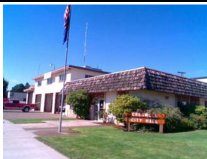
NE Vertical Irregularity Primary vertical irregularity is due to the fire station on the left side of the picture. Lane_pol04 is in the city hall building on the right side of the pic
