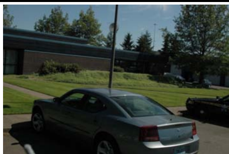
NE General Site bldg. on left
