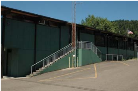
E Vertical Irregularity Primary a sloped site.
