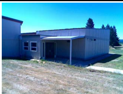
NW Plan Irregularity Primary Also shows a vertical irregularity.
