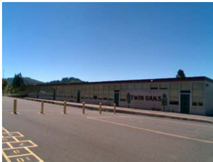
NW Plan Irregularity Tertiary Approximately 100 ft of windows with no apparent lateral system indicating a potential torsion problem.
