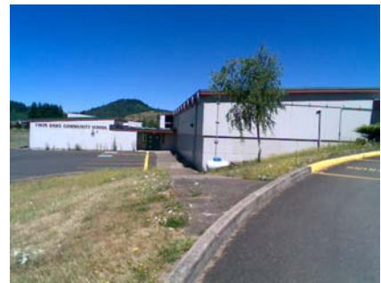
W Vertical Irregularity Secondary sloped site
