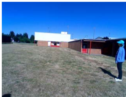
E Plan Irregularity Primary also shows vertical irregularity due to adjacent building. Building B is on the right and building C is on the left.
