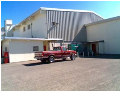
SW Plan Irregularity Primary The smaller building on the left is RM1 and the others are Concrete w/ S3.
