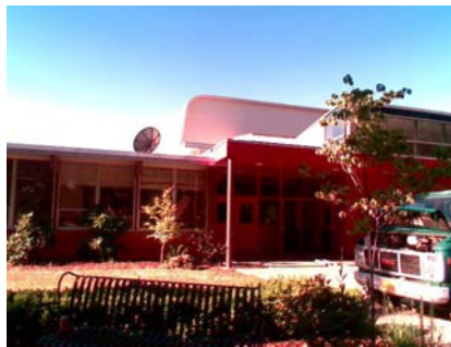
N Vertical Irregularity Secondary building B is shown on the right and building A is shown on the left.
