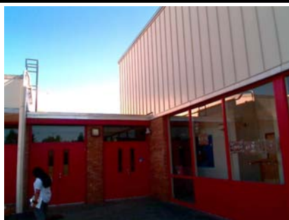
SW Plan Irregularity Primary also shows vertical irregularity due to adjacent building. The top half is S3 and the bottom half is less clear.
