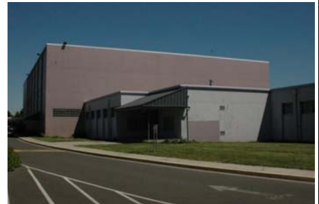
SW Vertical Irregularity Primary also shows reentrant corner
