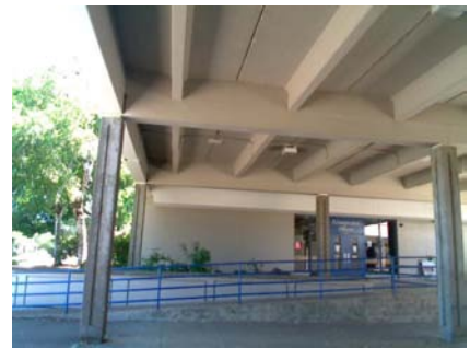
S Primary Structural Type Precast T beams and Precast Frames with a RM wall in the background.
