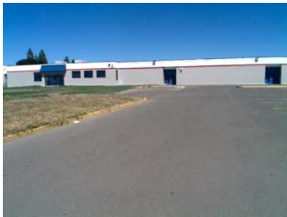
W Plan Irregularity Primary out of plane lateral system due to building C on the left (small reentrant corner due to adjacent bldg).
