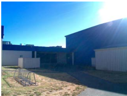
SW Vertical Irregularity Primary Also shows plan irregularity due to adjacent building.
