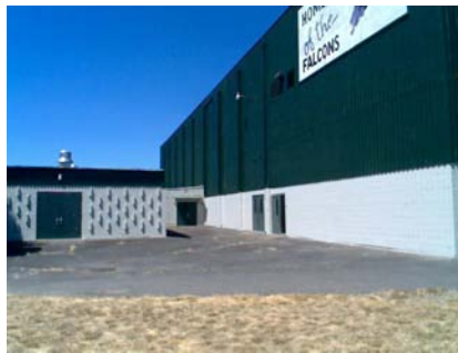
SE Plan Irregularity Primary also shows vertical irreg.
