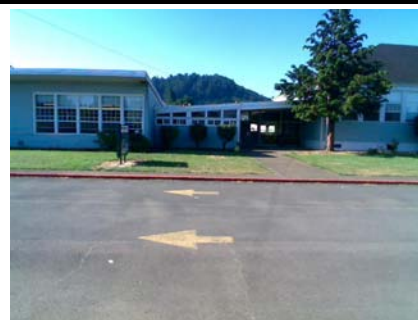
N Vertical Irregularity Primary also shows plan irregularity due to building A
