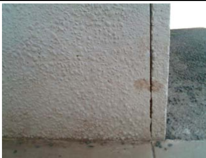
E Primary Structural Type 4 in thick concrete wall
