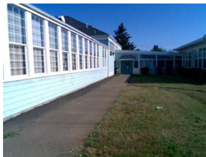
SE Vertical Irregularity Primary irregularity due to building addition.
