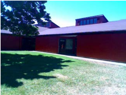
E Plan Irregularity Primary minor opening in the roof diaphragm
