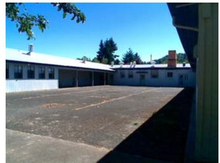
W Plan Irregularity Primary also shows a URM chimney
