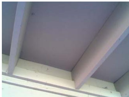
W Falling Hazard rafter toe-nailed to ledger
