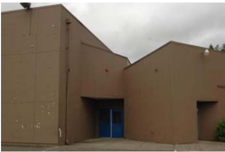
S Vertical Irregularity Primary Due to adjacent building, building A is in the right and building B is on the left.
