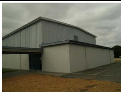
E Primary Structural Type and secondary structural type. W2 on the upper level and RM1 on the lower level
