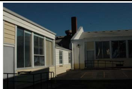
SE Falling Hazard Also shows a reentrant corner.
