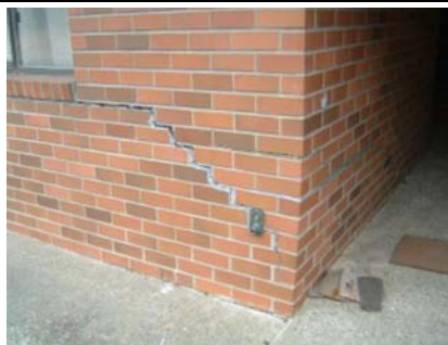
NW Poor Condition cracks
