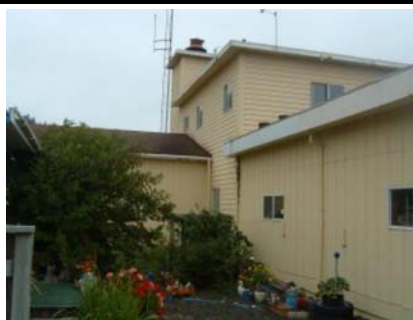
NW Plan Irregularity Tertiary step in elevation also
